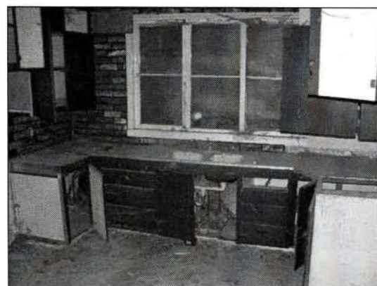
Figure 9. Interior View of Kitchen Area.
