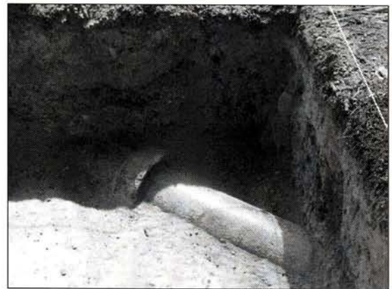
Figure 14. Drain Pipe Connecting to Southeast Corner of Foundation.
